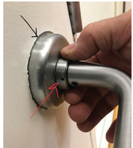
Figure 14. The black arrow points to the paint removed by the movement of the rosette. The red arrow points to what Best refers to as the "rose ring."
