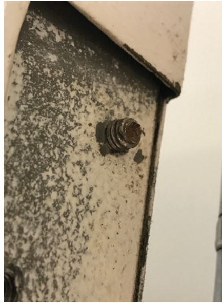
Figure 7. The author used needle-nose pliers to back out the screw.
