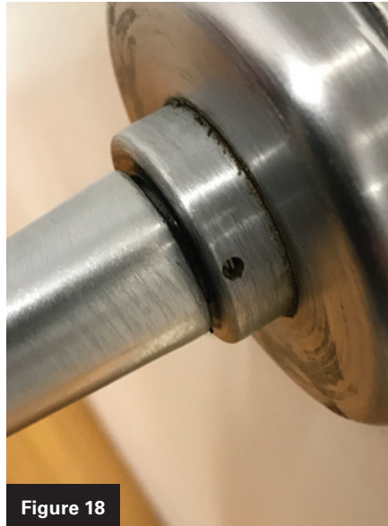
Figures 17 and 18. The rose ring is shown before and after tightening. Note the gap between the lever and the rose ring.
