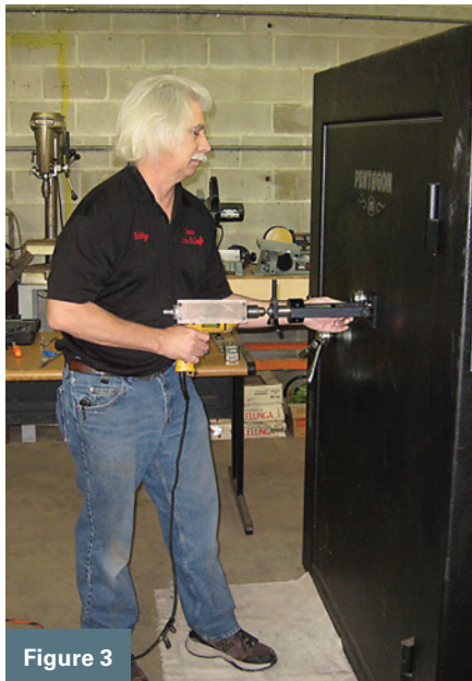
Figures 3 and 4. After a malfunctioning flex scope kept him from using the hole he had drilled in the side, the author ended up front drilling it and scoping the fence.
