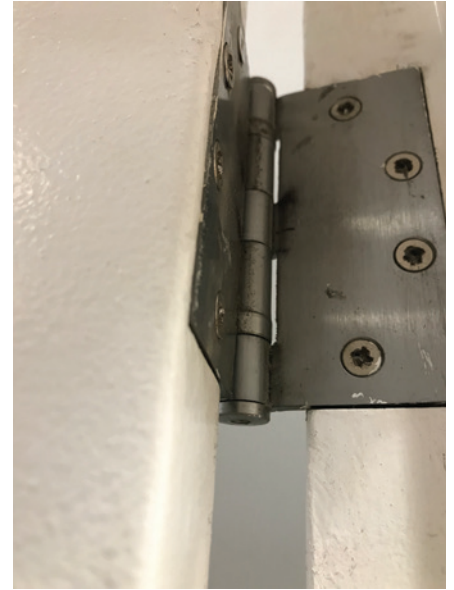
Figure 8. The hinge leaf is flush with the door.
