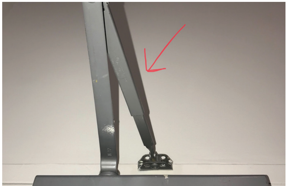
Figure 10. The arrow is pointing to the arm attached to the frame. This arm — and not the other — should be perpendicular to the closer body.
