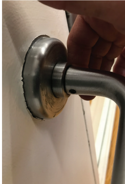
Figure 16. The author is lifting his finger so you can see the wrench hole isn't there anymore. Therein lies the problem.
