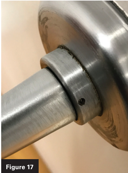
Figures 17 and 18. The rose ring is shown before and after tightening. Note the gap between the lever and the rose ring.
