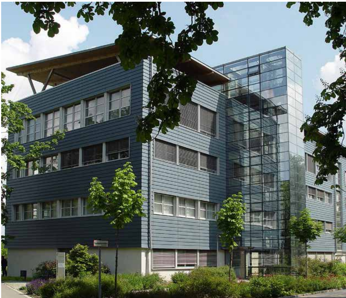
Anhalt University Campus Building at Bernburg
