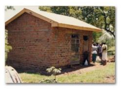
Figure 15. Mushroom house made of earthen bricks, cement walls and iron sheet roof.
