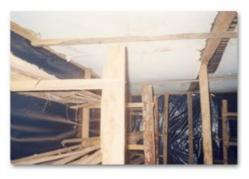
Figure 12. Roof insulated with cartons
