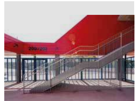
Stairs to the second level of the Grandstand.
